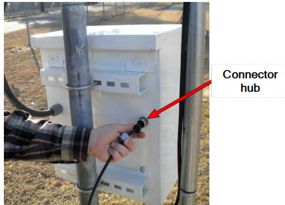
Figure 43 – Feeding Conductor Wire
