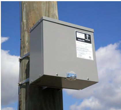
Figure 67 – UPS Attached to a Large Pole
