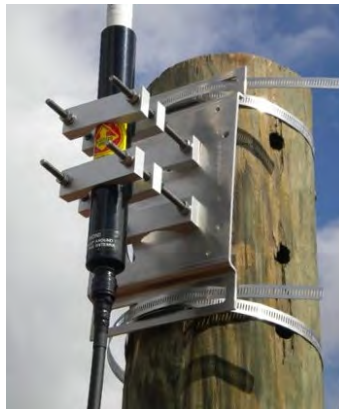
Figure 55 – Weatherized Connection
