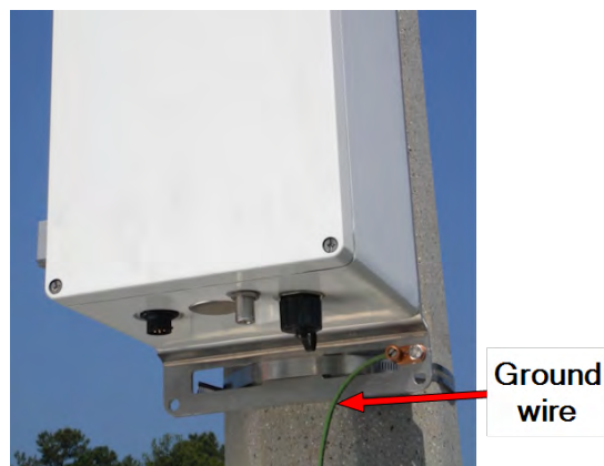
Figure 46 – Ground Wire
