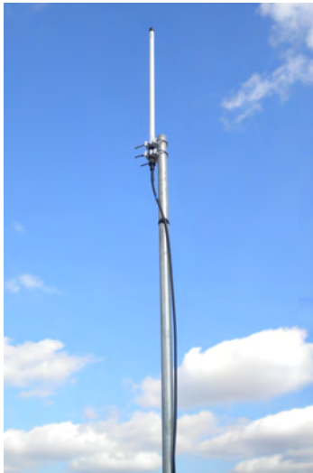
Figure 85 – Securing the Coaxial Cable
