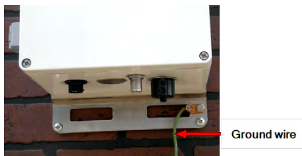
Figure 74 – Ground Wire
