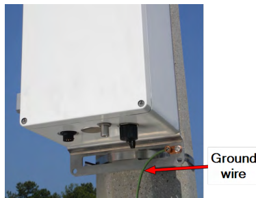
Figure 63 – Attach Ground Wire
