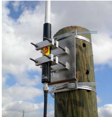
Figure 54 – Coaxial Cable Attached
