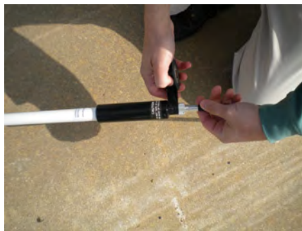
Figure 32 – Weatherizing the RF Antenna
