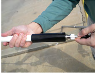
Figure 31 – Attaching the Coaxial Cable
