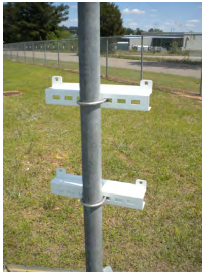
Figure 34 – Installing Pole Brackets
