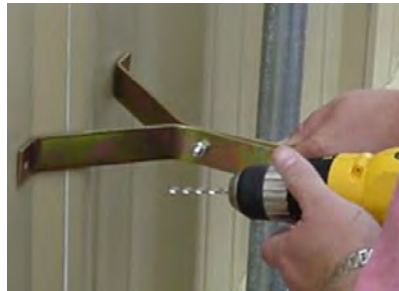
Figure 80 – Lining up Second Pole Bracket
