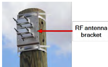
Figure 52 – Large Pole Bracket
