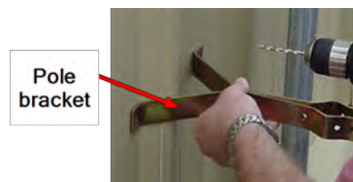
Figure 79 – Securing Pole Bracket
